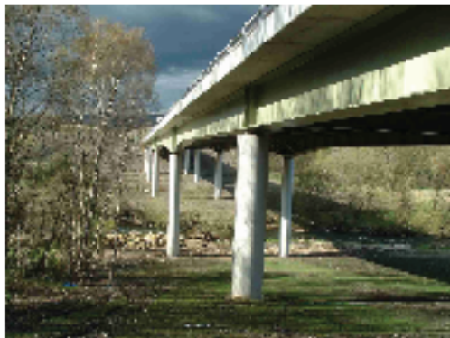
Bingley Bypass Viaduct spanning the River Aire
